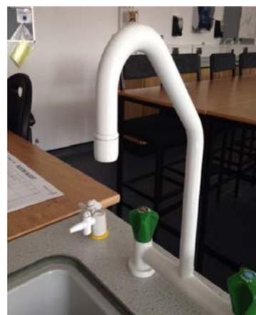
Figure 6: non convulsive hose union taps (sometimes called hoseless taps) must be fitted in Fig 3: Scenario B – rooms 2, 3, &4. The tap gap must be maintained at all times
