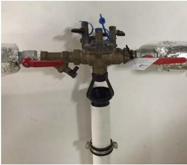
Fig 10: reduced pressure zone (RPZ) valve
