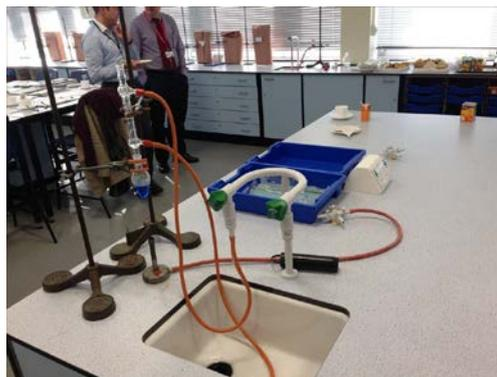
Fig 7: attaching laboratory equipment to lab tap compromises the "tap gap" – backflow protection is required e.g. supply from a storage cistern
