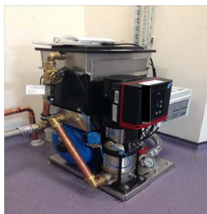
Fig 2: Storage cistern (break tank) supplying school laboratory
