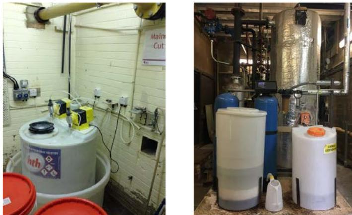
Fig 15: examples of equipment found in swimming pool plant rooms.
